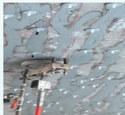
RC床版のひび割れ補修
